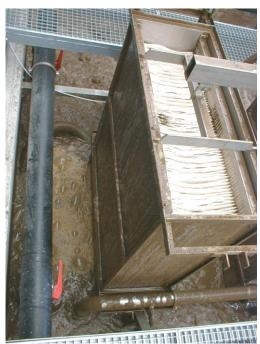
The recent development of membrane bioreactorsystems (MBR – see http://www.envicare.at/research/kommeng.pdf, Lit. 2 - 5) seems to be very promising to reduce the amount of the "secondary" sludge. These systems operate with a dry solids concentration from 8 – 20 g/l and ensure an aerobic stabilisation during the treatment.
