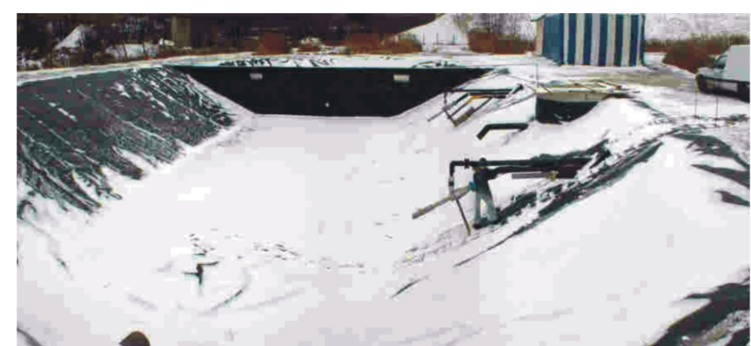
Two ponds have been put out of service, the remaining lagoon has been equipped with an ejector aeration system.
