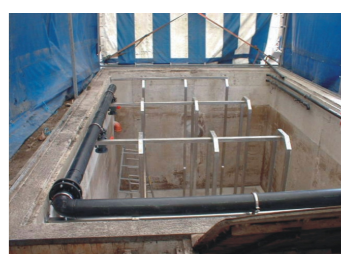
The WWTP has been equipped with a MEMJET membrane filtration system.
