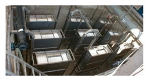
The basin is due to of technical matter constantly aerated by the coarse bubble system.
