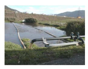
First of all the original wastewater plant, built in 1989 as a ventilated pond purification plant (see left pic.), had to be converted. Two of the three existing lagoons were put out of service, while the remaining lagoon was equipped with a ejector aeration system and a partition wall to create a separate settling basin. In this area sludge is collected and recirculated, the excess sludge is removed with the primary sludge.
