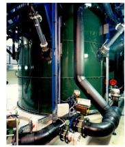
halogenated hydrocarbons are converted to gaseous carbon dioxide and nitrogen with the help of bacteria. In order to cope with the great contaminant load, the unit must contain large quantities of bacteria, namely 20 to 30 g/L, which is seven times more than is contained in a conventional sewage purification plant.
