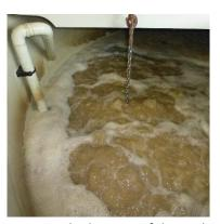
The biological treatment takes place in the MBR tank. Due to the membrane, all biomass in the form of activated sludge is held back and therefore, the sludge age can be freely chosen. Aer-
